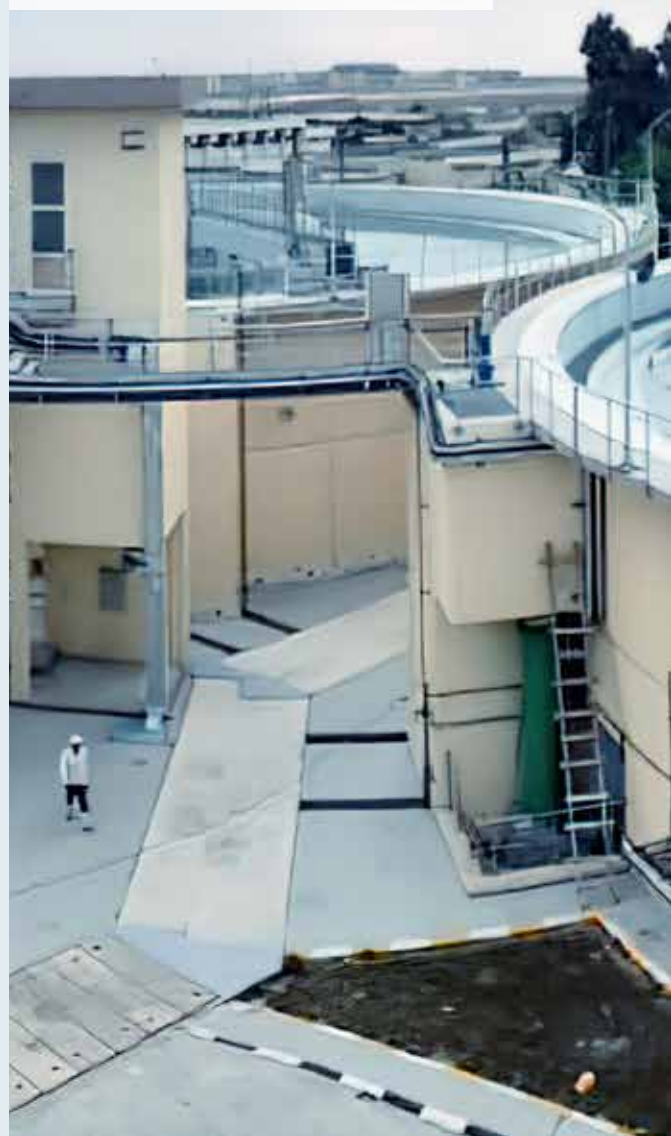
El Raswa WTP II, Port Said, Egypt: multi-stage system for treatment of Nile water, 80,000 m³/d
